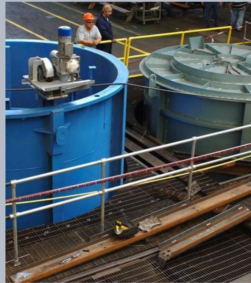
TEMPER TANK AND FURNACE HI-TECH
